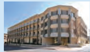
AMICAVILLA INAGE (HCM)
