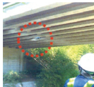
Bridge inspection using a drone in progress
