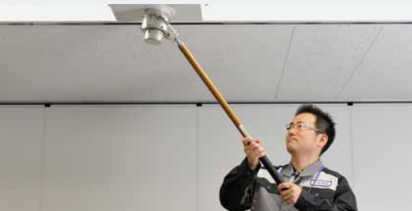
Inspection of fire extinguishing equipment
