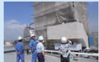
ALSOK BUILDING SERVICES employees explaining progress of large-scale renovation project
