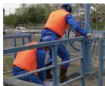
Sluice pipe operations
