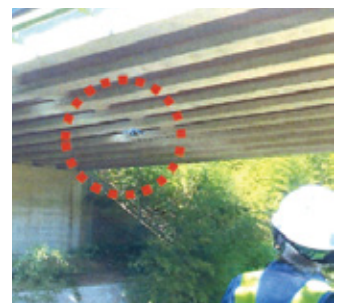
Bridge inspection using a drone in progress
