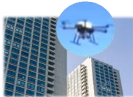
Exterior wall investigation
