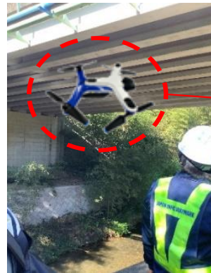
Bridge inspection by drone
