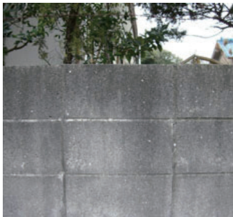
Before/洗浄後施工
